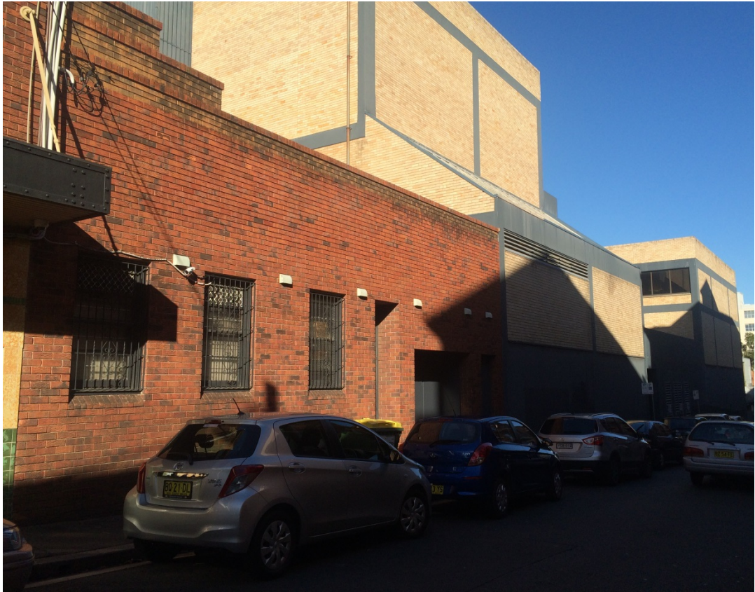
Figure 7: Existing single storey element at the rear of the Alfred Hotel
